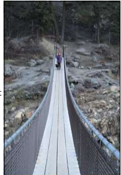
The swinging bridge.
